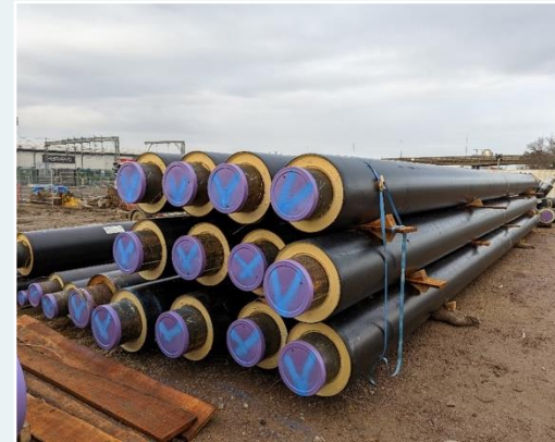
Pipework in storage
