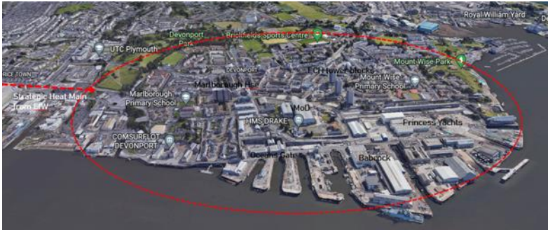
HNDU refresh/ Devonport Feasibility Study LA vision of heat off take expansion MoD site modernization Oceangate developments
